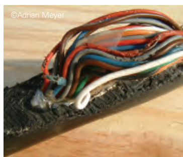
Damaged wiring can lead to fires
