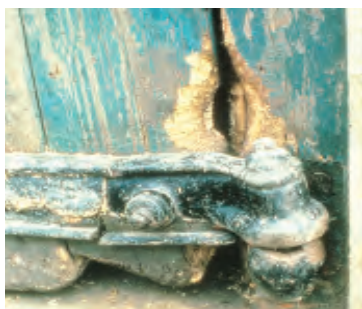
Building structures can be damaged
